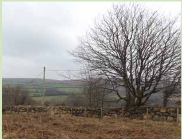
The rebuilt stone wall
