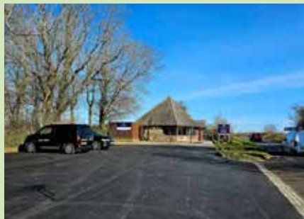
The new surface on the car park
