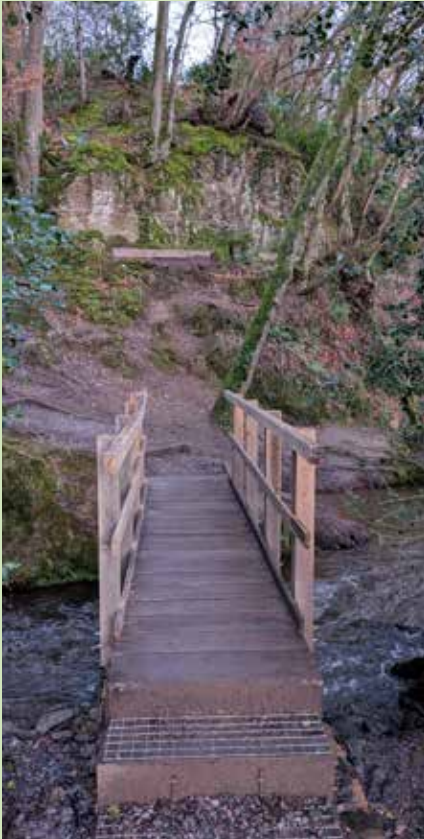
The new footbridge
