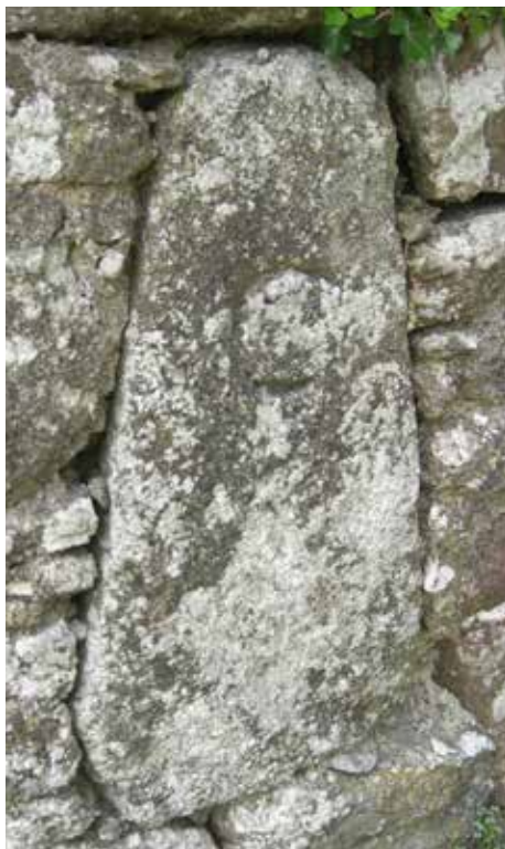
Ponsworthy Bridge 'C' Stone, North
