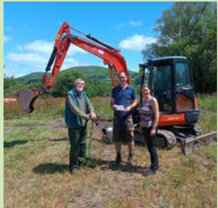
Digging the turf for the start of the building work Widecombe Community Hall
